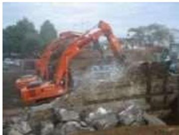
Demolition of redundant two lane solid concrete and steel constructed rail over bridge in Papakura. Successfully completed within a 24hour timeframe.
