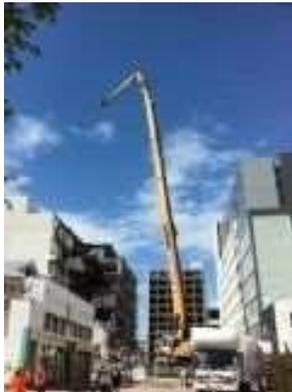
The largest high reach excavator in the Southern Hemisphere, Twinkle Toes is finally in Christchurch to assist with the recovery to rebuild by providing safe, fast and efficient deconstruction options for buildings in excess of 10 storeys.
