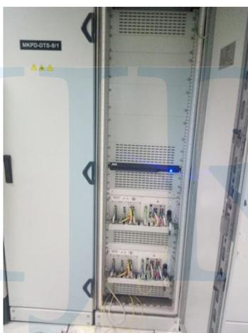
Fig4. Computer based interlocking unit (CBI)
