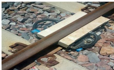
Fig5. Axial counter on track with transmitter and receiver connected via fibre optical cables.
